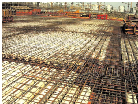
Fig. 4. Cast-in-place hollow-core slab in practical engineering
